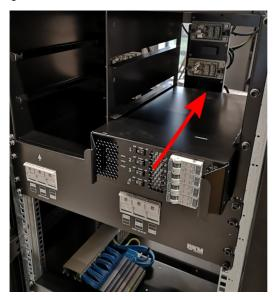
NOTE! Make sure the modules are fully inserted.
