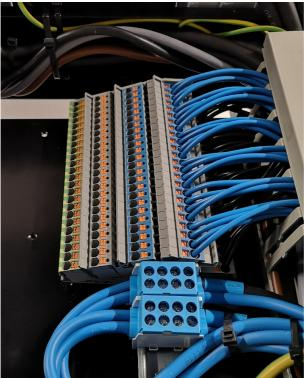
**NOTE!** The phase, neutral and ground wires of one receiver must be connected to the same terminal group.
