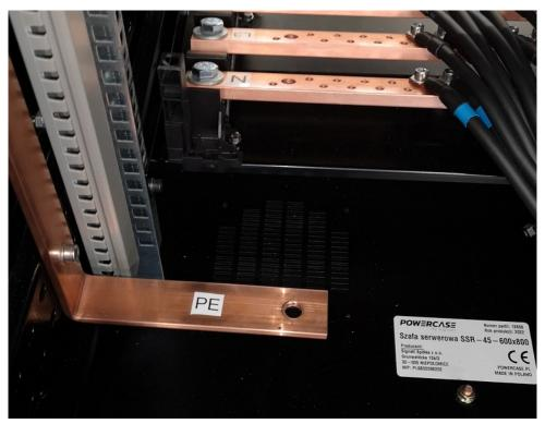
The screw must be tightened with a force of 50Nm. The cable must be equipped with a cable lug for an M10 screw. *An M10 screw is included*.
